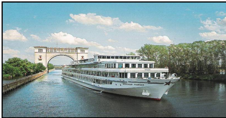
Photo 1: An Example of Lock Elevation from Uglich
